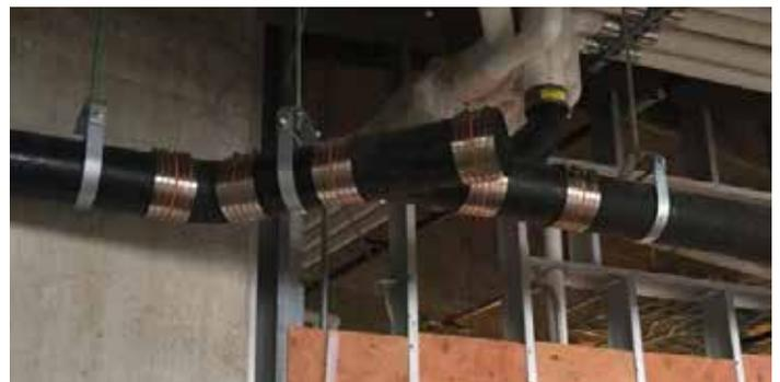
Sporting venues present many challenges as multiple contractors are working in the same space simultaneously. That's why pre-planning, prefabrication and computer modeling were critical to the arena project helping to keep us stay in front of the construction schedule. Pre-assembly of cast iron plumbing systems joined with heavy-duty couplings improved our efficiency with greater accuracy.
