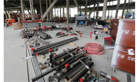
"By using cast iron piping materials along with the Husky couplings, we are able to air test the system at our manufacturing facility and then transport the complete plumbing systems to the building site without the worry that there would be joint failure.
